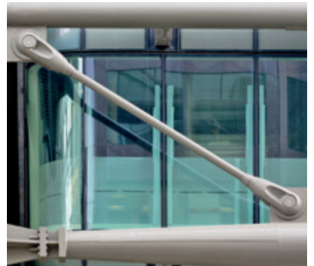
ASD0540-S tie bars M76 to M160 were used as the tension elements in the trusses to form part of this unique and structurally demanding London office building at Cannon Place.
