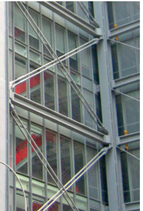
Tandem ASD0540-S bars were used to brace the new 52 floor headquarters for the New York Times newspaper.
